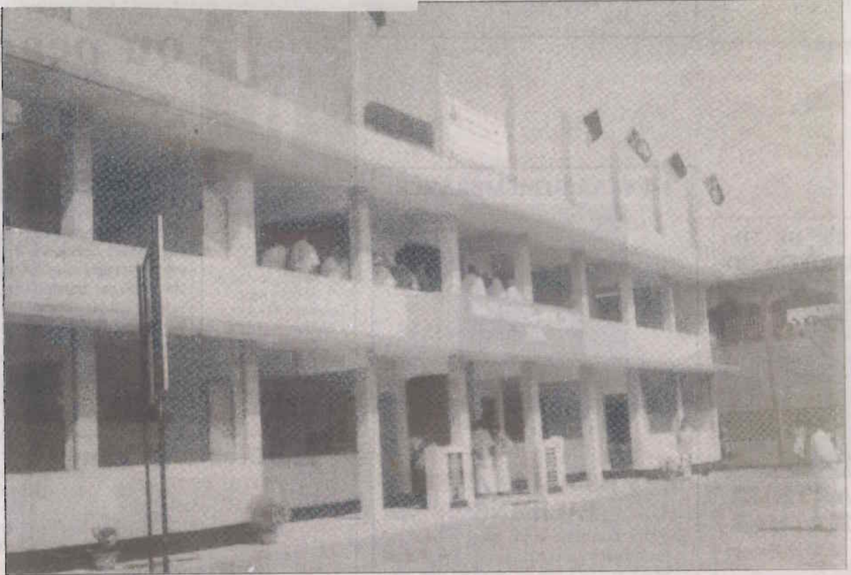
NEW BUILDING: The new two storey-building at Naleem Hadjar Ladies College which was opened by Karl Eyarkauer - the Former District Minister of Main-Kingzing-Kreis-Germany recently at China Fort, Beruwala. (Pic by M. B. M. Mukthar)
